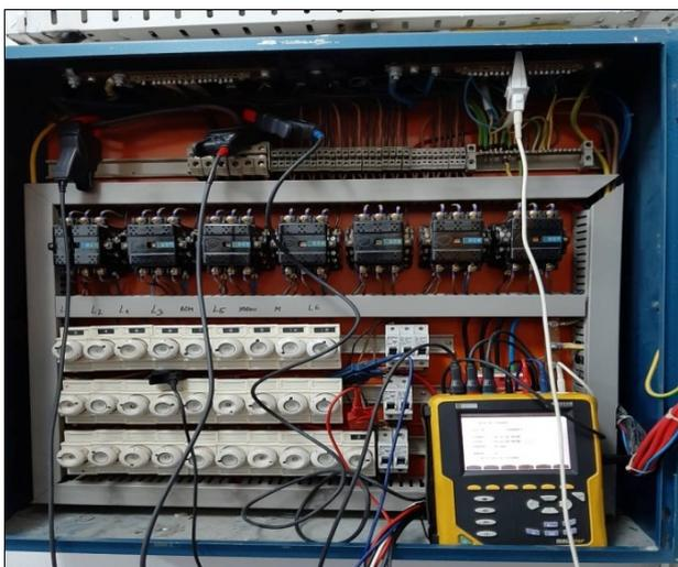
Fig. 1. Photo of measurement location during measurement at the computer centre
