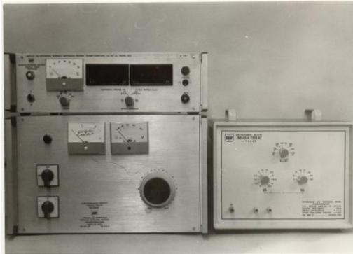
Fig. 10 System for voltage transformers accuracy testing, type NIT-2p (1981.)
